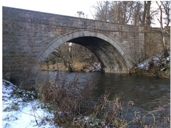
Figure 5-14: Bridge with Negligible to Low BRP. See Target Note 5. Photograph taken 30 November 2017 15:23 Photograph location: NJ 78270 20490
