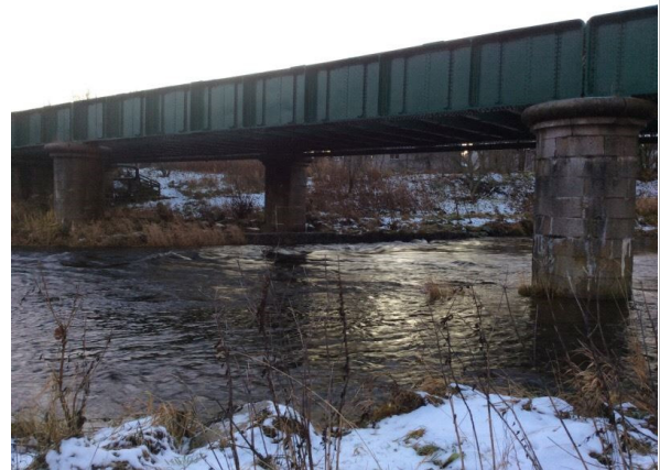
Figure 5-2: Rail bridge with Low BRP and Giant Hogweed at base. See Target Note 9 Photograph taken 30 November 2017 15:41 Photograph location: NJ 78108 20079
