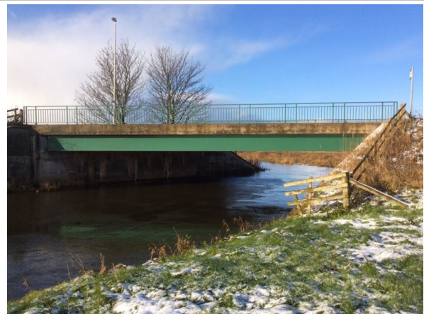
Figure 5-4: Bridge with Negligible BRP. See Target Note 1. Photograph taken 30 November 2017 11:37 Photograph location: NJ 77979 22155
