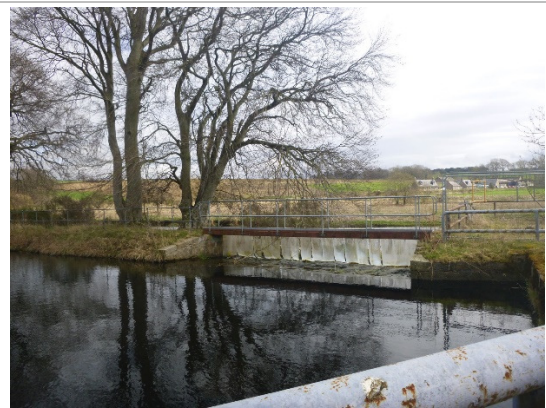
F: Sluice leading to weir at downstream extent of the canal/ mill lade at Kirkwood Commercial Park. (OS NGR NJ 78282 19168)
