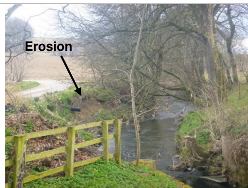
B: Downstream from Lethenty House, erosion visible on left bank near an outlet pipe. (OS NGR NJ 76958 24629)
