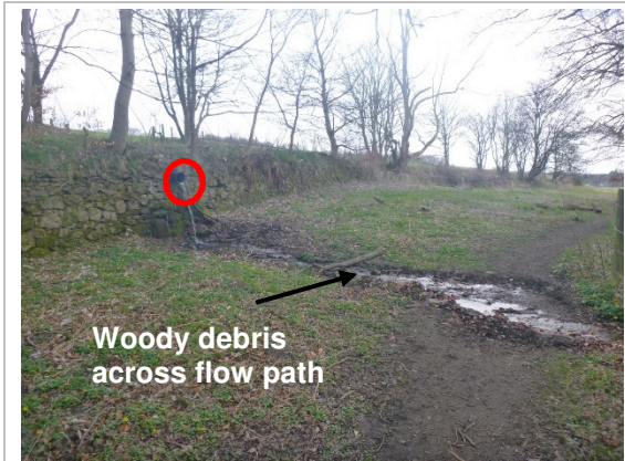
C: Outflow pipe discharging and creating a channel towards the Don across the public footpath. Slowing this outflow and channel formation recommended. (OS NGR NJ 76376 20204)
