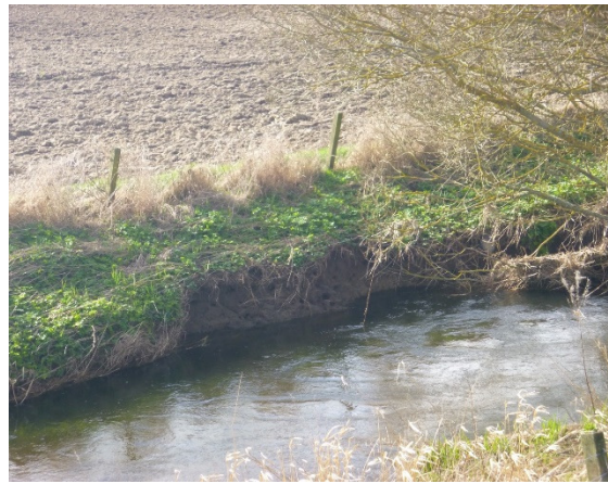
F: Bank erosion causing instability upstream of the Ton Bridge. (OS NGR NJ 71512 14650)
