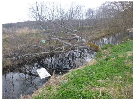
H: Natural and man-made debris in the canal. (OS NGR NJ 77945 20166)
