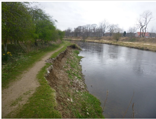
C: Significant bank erosion below the footpath on left bank of River Don. (OS NGR NJ 77906 20418)
