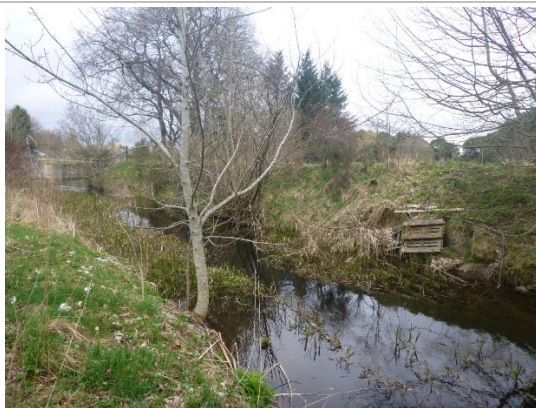
E: Canal by Port Elphinstone with embankments on both sides, stagnant water and debris input. (OS NGR NJ 77796 20434)
