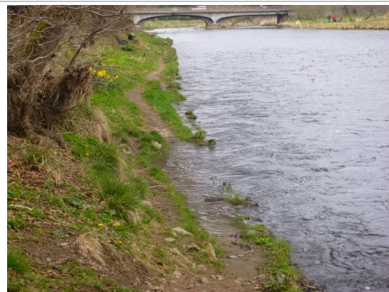
F: Eroded footpath along left bank of Don south of the A92 road bridge. (OS NGR NJ 77403 20593)
