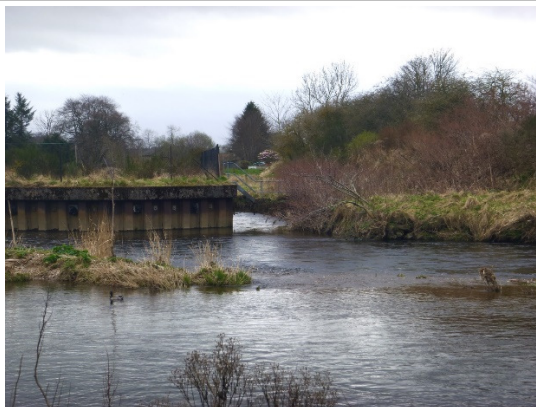
G: Entrance to the Old Canal on the right bank of the Don and erosion on the right bank. (OS NGR NJ 77685 20648)
