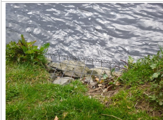
G: Gabion basket lining the eroding left bank of the Don downstream of the B993 road bridge. (OS NGR NJ 77490 20616)
