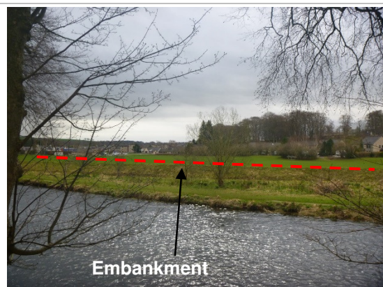
H: Embankment along Davidson Field playing fields. Works to reinstate the crest were carried out following the last large flood event. (OS NGR NJ 77490 20616)
