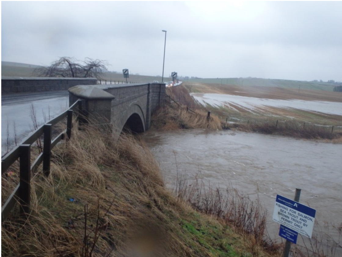
B9001 Howford Bridge (north of Inverurie on the River Urie) @ 14:37
