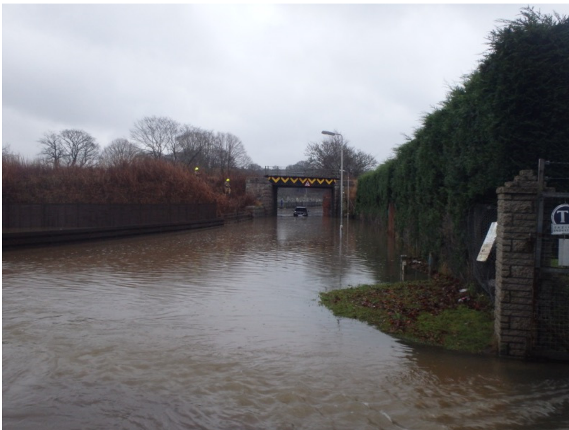
Car stuck under Port Elphinstone Rail Bridge on B993 Keithhall Road (near WwTW) @ 14:10
