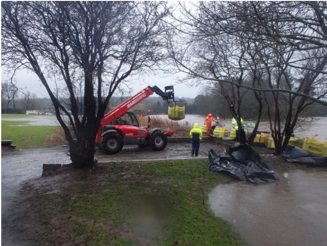
Adjacent to Inverurie Precast, River Don upstream of Broom Inch (flood wall built by Precast to protect property) @14:15
