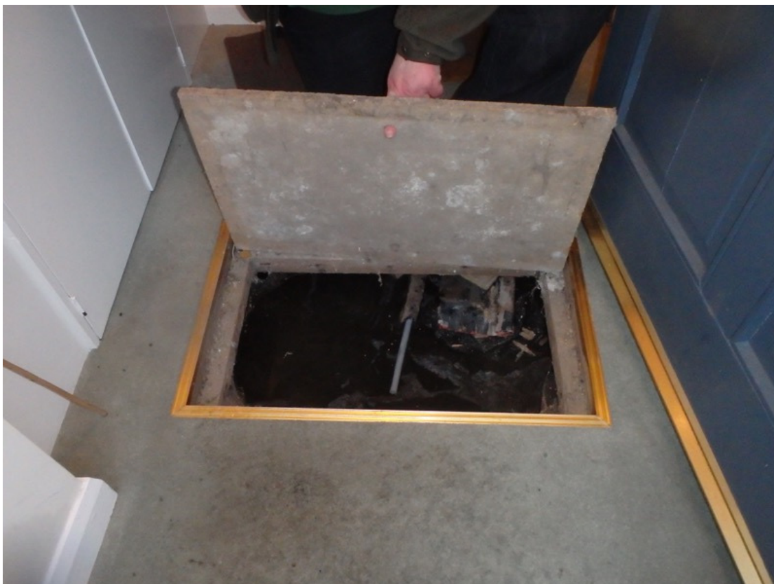
Basement of property on Canal View @ 15:30
