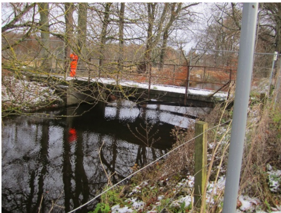
Upstream view of bridge
