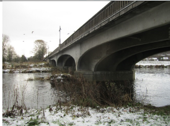
View from downstream
