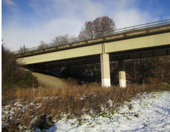
Upstream view of bridge
