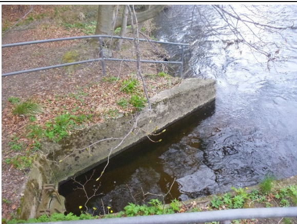
View of outfall and wingwall looking downstream
