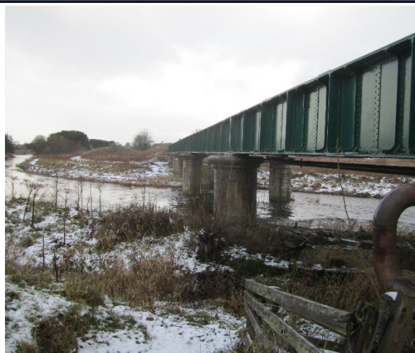
Upstream view of bridge
