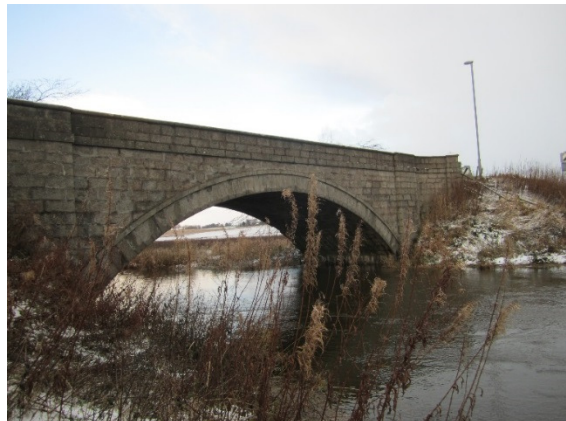
Downstream face of bridge
