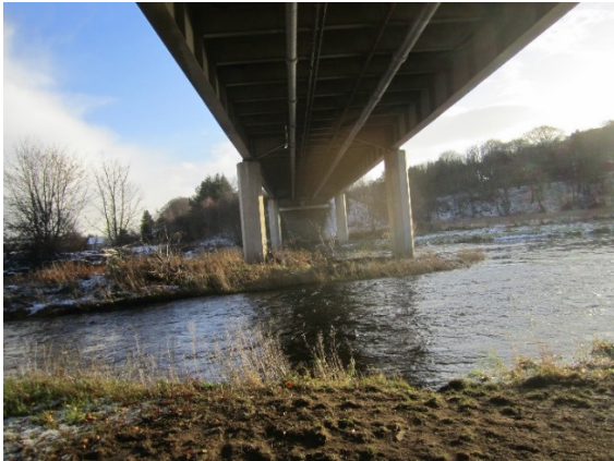
View of bridge from underneath
