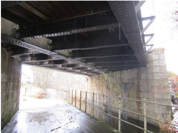
View from underneath
