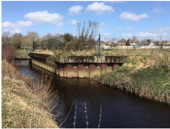
Upstream view of wall
