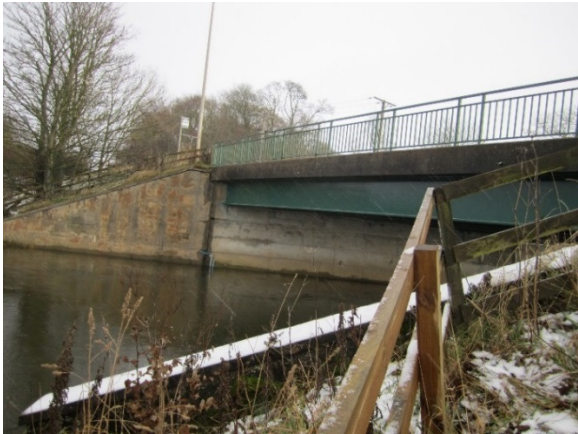
Upstream face of bridge, left abutment
