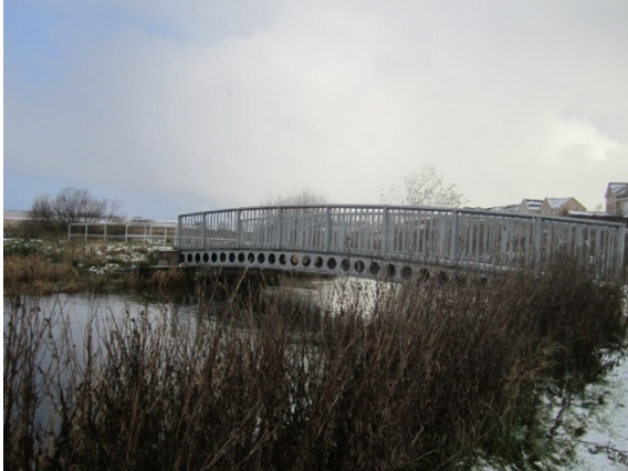
Downstream face of Footbridge
