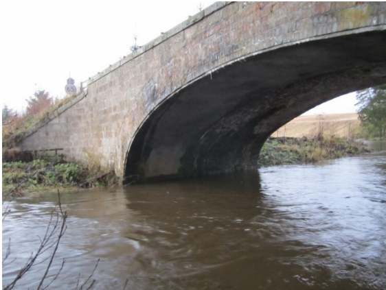
Upstream view of masonry bridge
