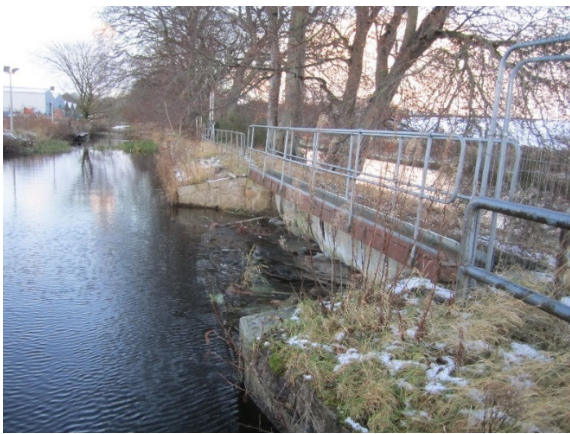
View from downstream
