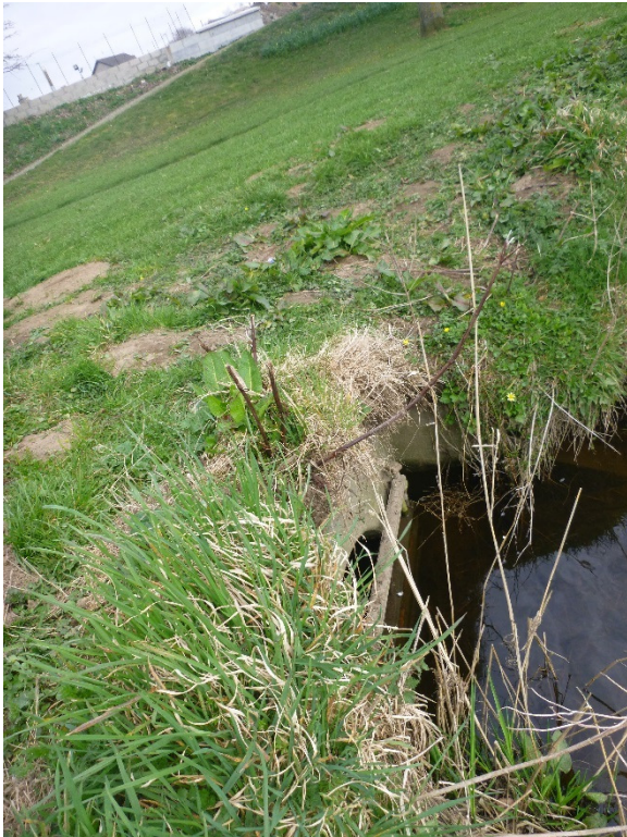
View of outfall
