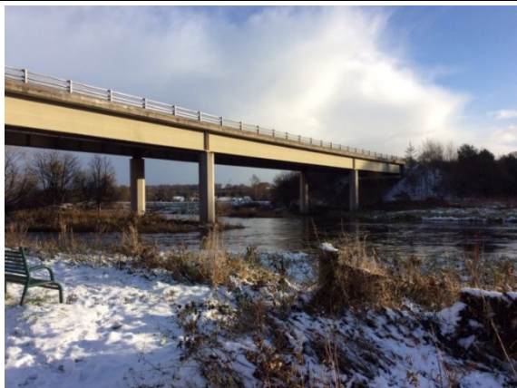
Upstream view of bridge
