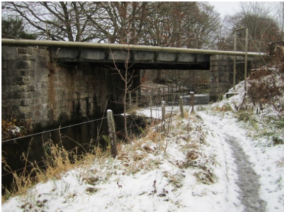
Upstream view of bridge
