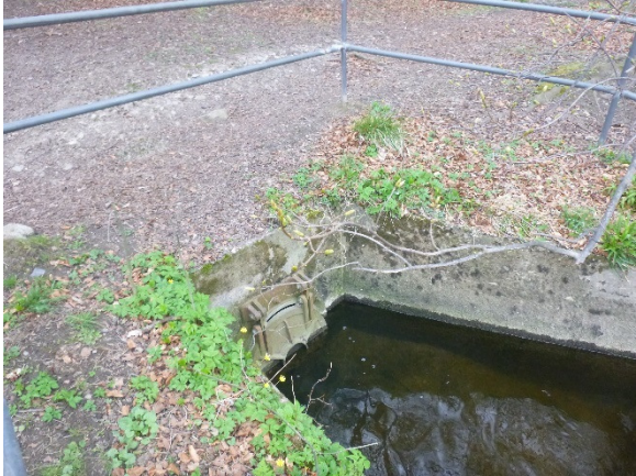
View of outfall and flap valve
