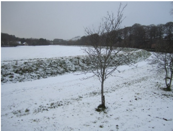
View from downstream
