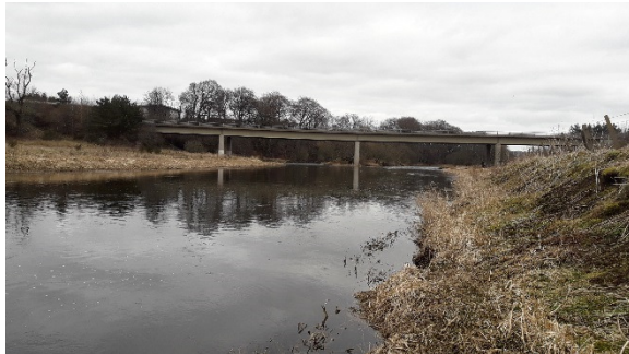
Area where the outfall should be
