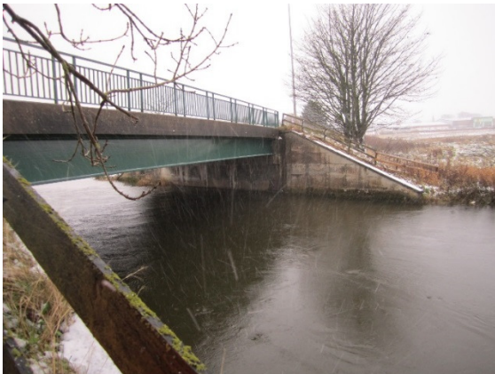
Upstream face of bridge, right abutment
