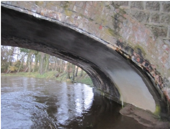
Upstream view of arch soffit
