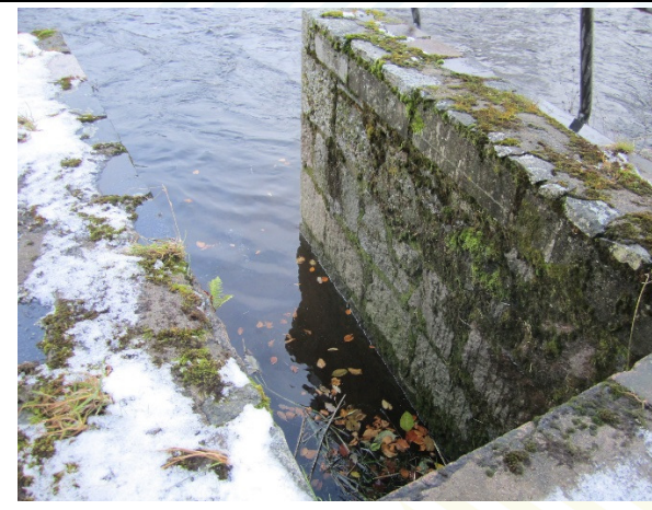
Outfall side walls
