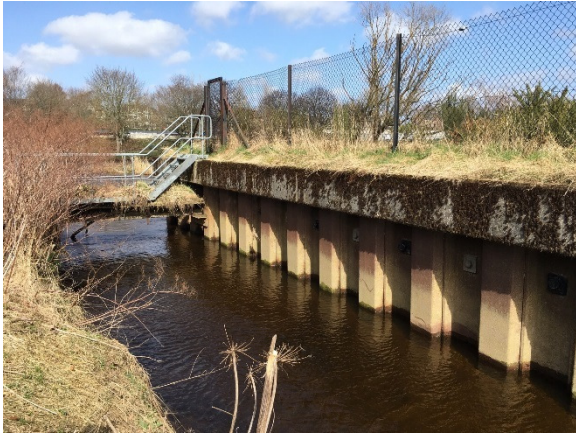
View of bridge
