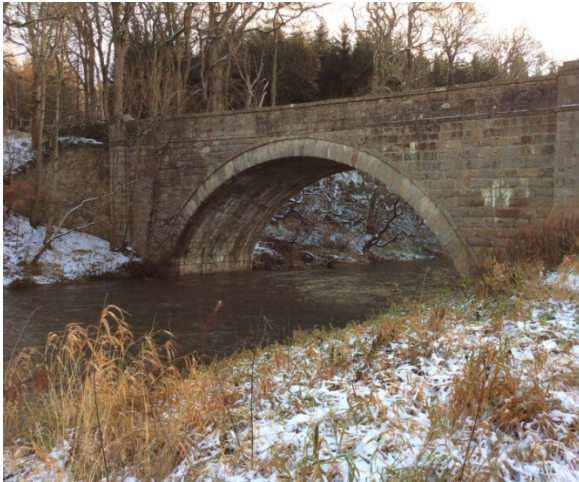
Upstream view of bridge
