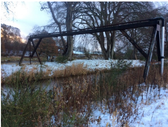
View from downstream
