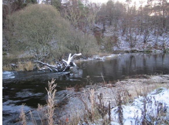
View of Weir
