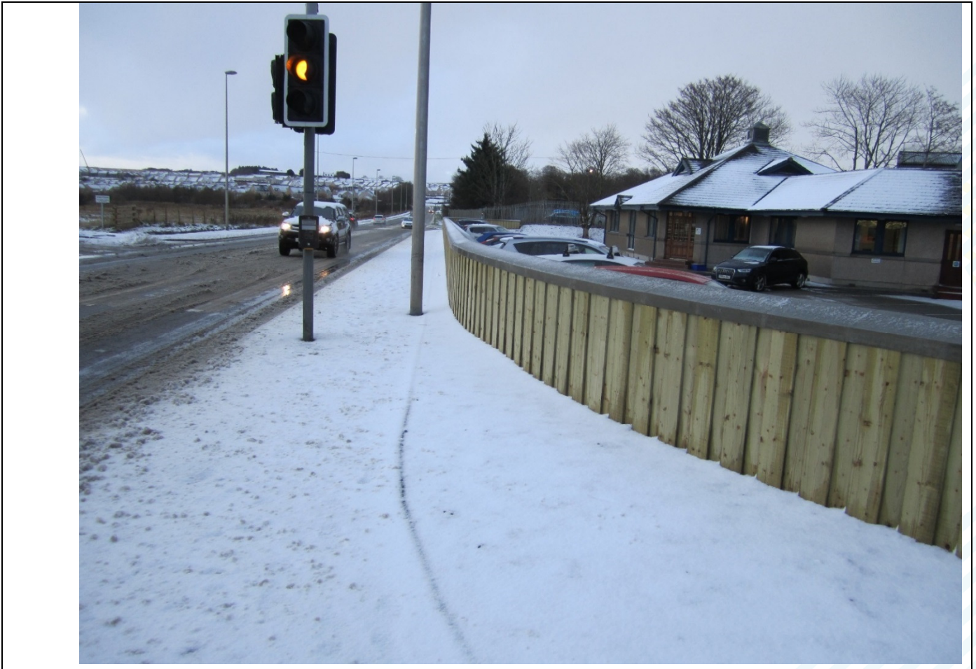
Figure 5-4: Property Level Protection of commercial property (Scotframe Timber Engineering Limited) off B9170 (No. 2)
