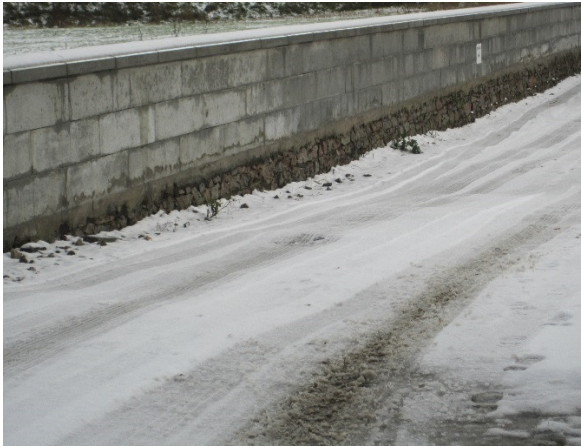
Left hand side of the wall
