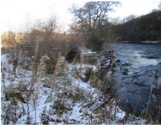
Upstream view of sluice gate
